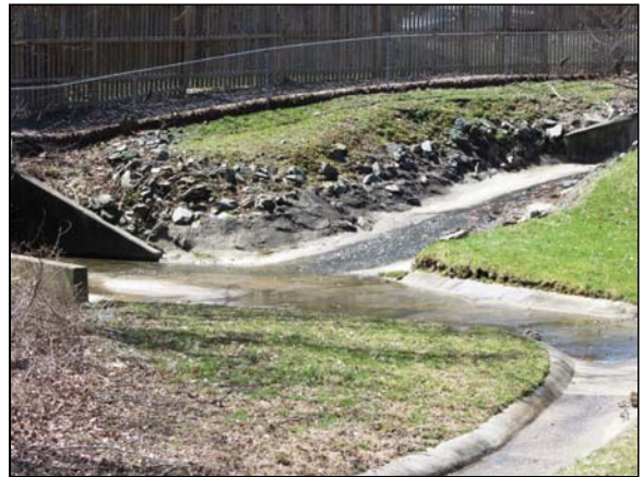
Photo #58. Trickle ditches in the stormwater impound facility.
