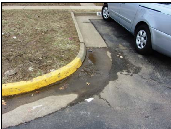
Photo #5. Typical depressed pavement and concrete curb & gutter may indicate damage to base materials and bearing soils beneath the asphalt pavement.
