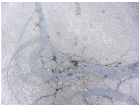
Photo #11. Crack sealing of alligatored pavement, typical.
