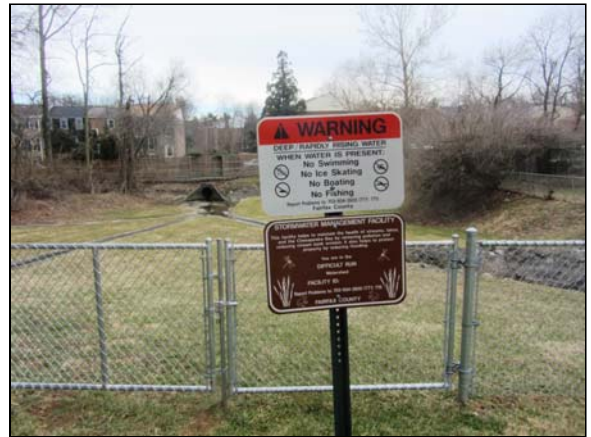
Photo #34. Signage at the impound facility.
