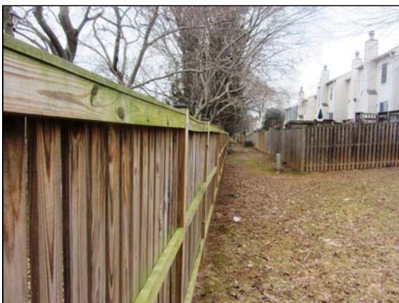
Photo #23. Wood stockade fence installed along the south property boundary.
