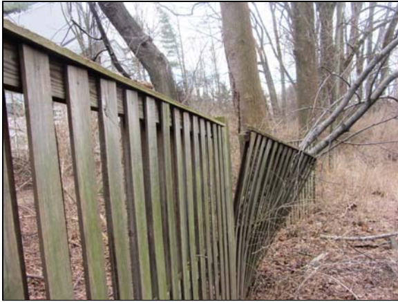
Photo #21. Fence installed along the east property boundary.
